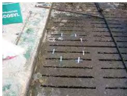
Figure 2 Separating a part of the slurry pit
